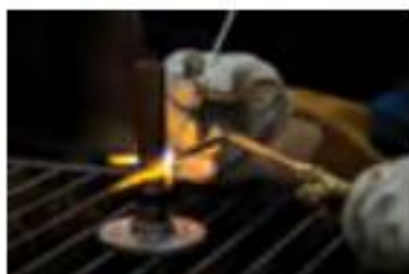
Oxy-acetylene welding 산소-아세틸렌 용접 Hàn acetylene-oxy
