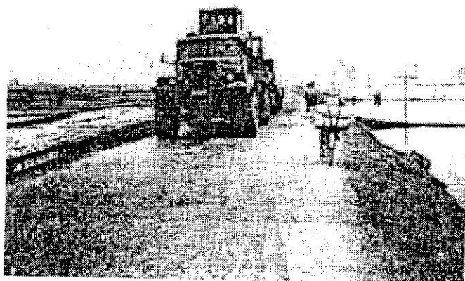
The growing number of heavy vehicles is putting extra strain on road structures
