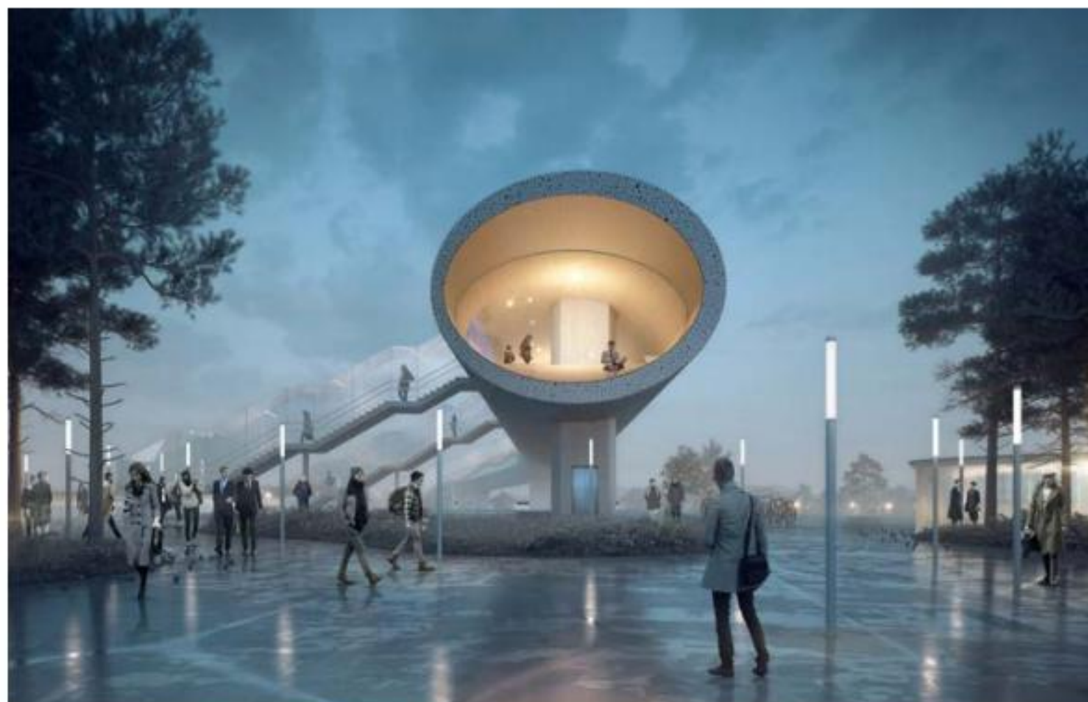
Køge North Station by COBE
