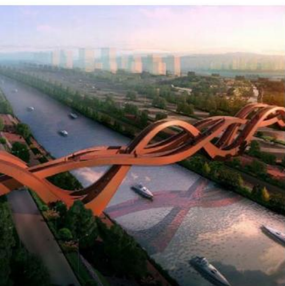
Lucky Knot Bridge by Next Architects
